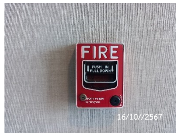
Fire Alarm Manual Station
